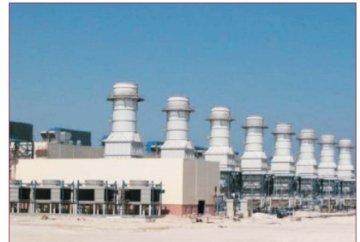
Figure 1: An open cycle gas turbine power plant, similar to the type to be constructed for this project.
